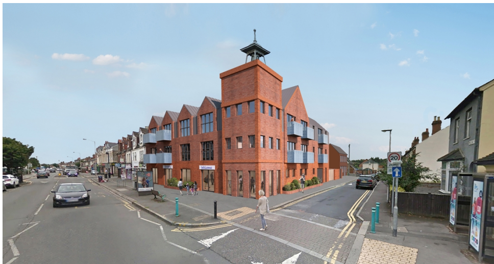
Balconies with glass
